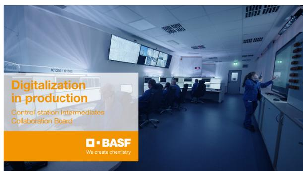
The modern control station in the intermediate products plant at the Ludwigshafen site is where all information relating to the plant comes together. Using numerous screens, the plant operators control and monitor the highly complex chemical processes.
